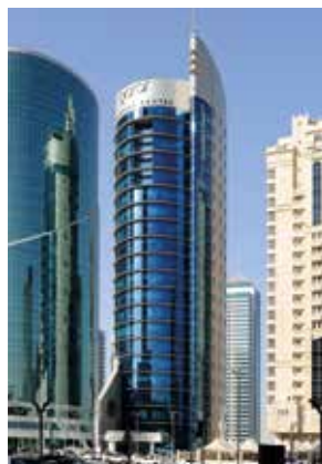
Doha, Qatar Financial Centre
